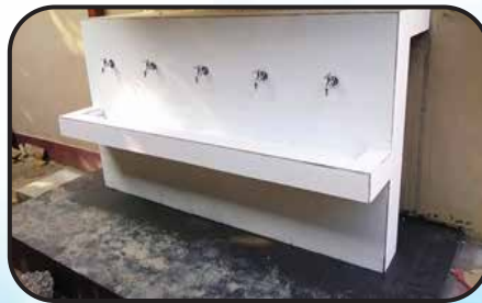
New water spot constructed at Navalkadu school
